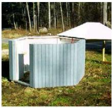
The structure is made primarily of 3 sheets of T1-11siding; three 3 sheets of 3/8-inch plywood for the roof; 10 fir 2x4s; 8 PT 2x4s; 6 (3/16xX2 inch) aluminum flat stock (bent to 25°); and one-half sheet of 3/4-inch plywood.
