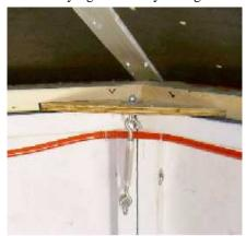
The roof is lightweight and supported to the rear by rollers made of sections of 3/4-inch conduit over a 1/2-inch conduit that acts like an axle. Cables loop around the supports, keeping the roof from falling to the side or blowing off in a gust of wind. A strap and hook arrangement holds down the lip when it rests on the back wall.
